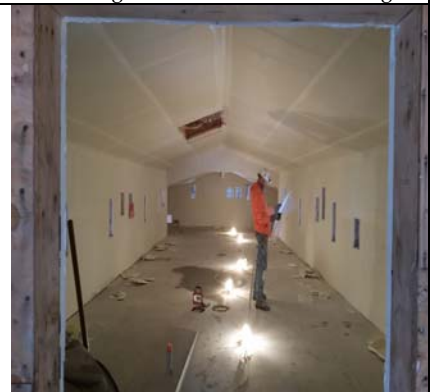
Mechanical Mezzanine Finish Progressing
