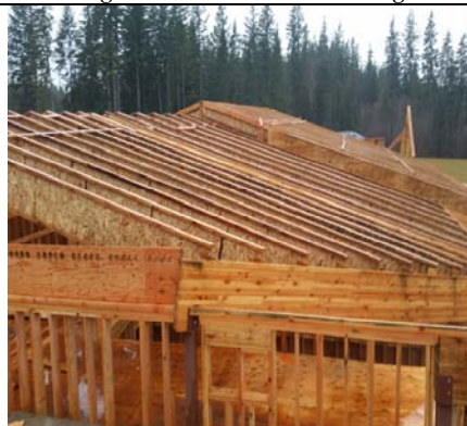
North Wing Trusses - Roofing Pending...
