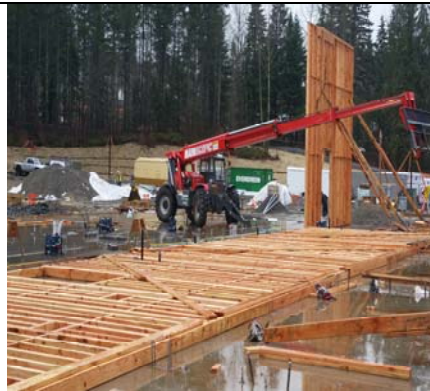
Administration Hallway Walls Framed
