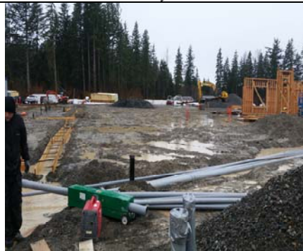
Stage/Multi-Purpose Area Footing Forms
