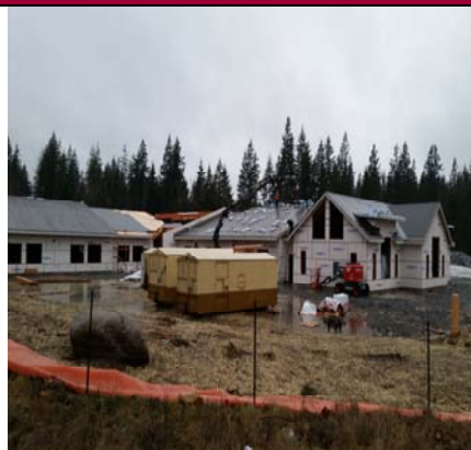
East Wing Weatherboard And Roofing
