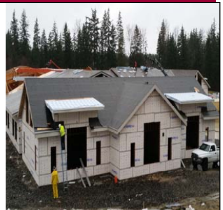
South Wing Weatherboard And Roofing
