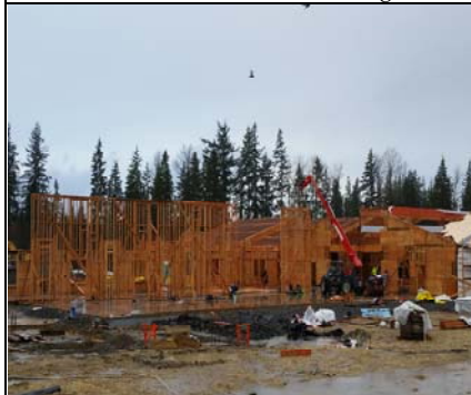
Setting Administration Hallway Wall
