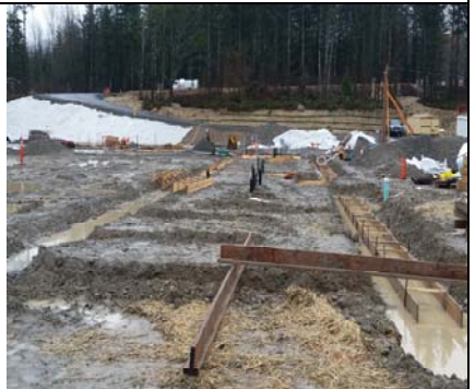
Restrooms/Kitchen Area Footing Forms
