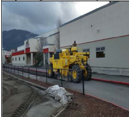
Front Parking Lot 3
