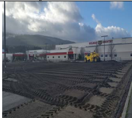
Front Parking Lot 4
