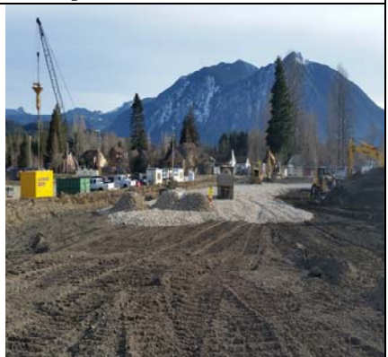
More Rock Pad For Stone Column Rigs
