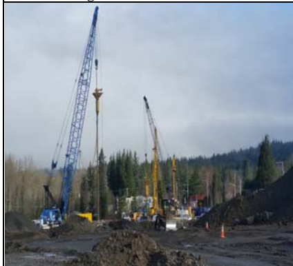
More Stone Column Installations
