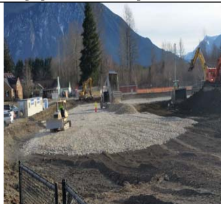
Bringing Grade Down Even More For Rock
