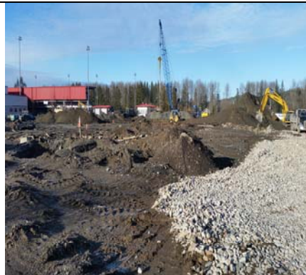
Bringing Down The Existing Grade
