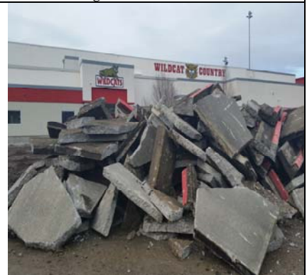
Concrete Sidewalk Demolition
