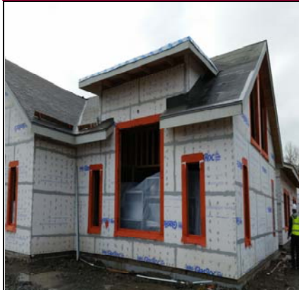
Building Dry-In With Window Wrap Prep
