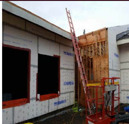
East-South-North Wing Connections Begin
