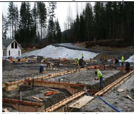
West Wing Footings Setup For Concrete
