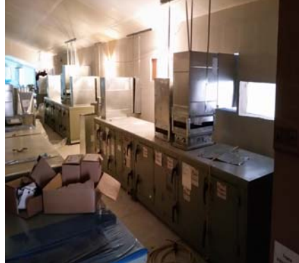
Heating/Ventilation/Duct Installation Begins
