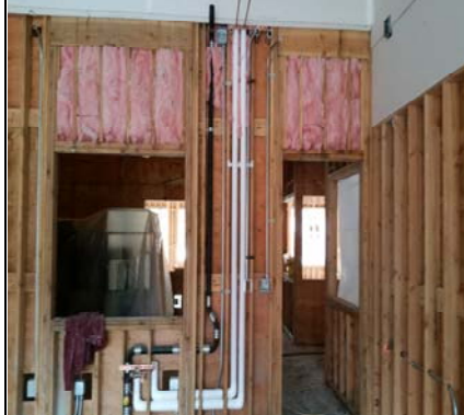
In-Wall Plumbing & Insulation Begins
