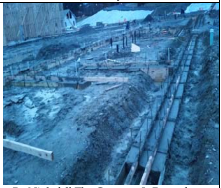
...By Nightfall The Concrete Is Poured
