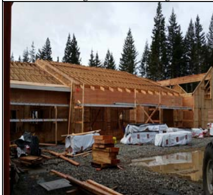
North Wing Trusses Ready For Plywood
