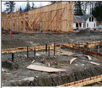
Looking At Gym Area Through Restroom
