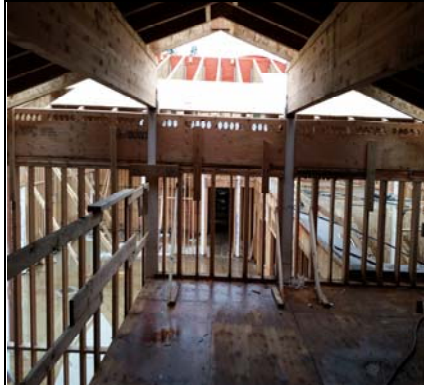
Roof Beam-Truss-Overbuild Tie-In Area
