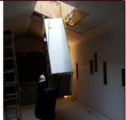
Receiving HVAC Units In Mezzanine
