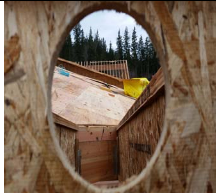
...More Roof Ventilation-Plywood-Trusses
