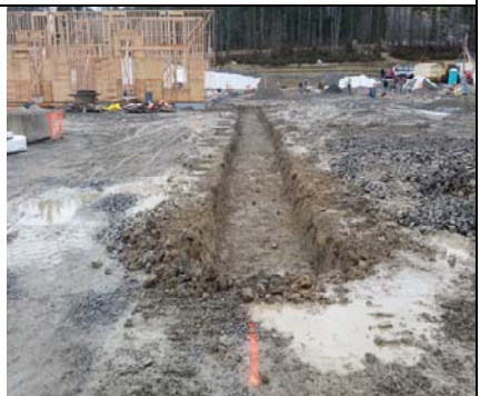
Gymnasium Area Pending Footings/Walls
