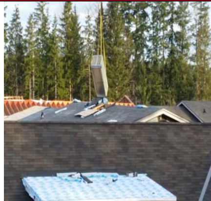
Crane Setting HVAC Units South Wing
