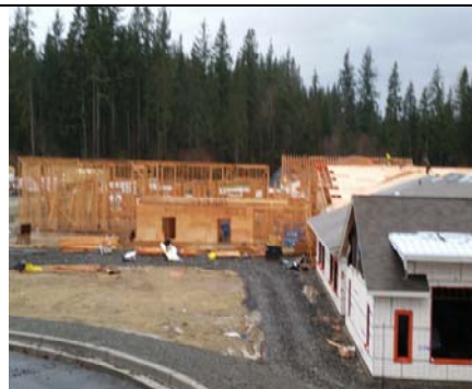
Administration Area Pending Roof Trusses
