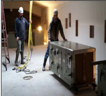
Dolly Rolling HVAC Units Into Position
