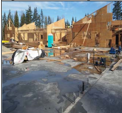
North Wing From Administration Area
