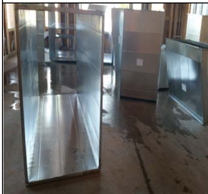
Large Ventilation Ductwork Begins
