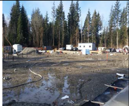
Multipurpose/Gymnasium Wing Pending
