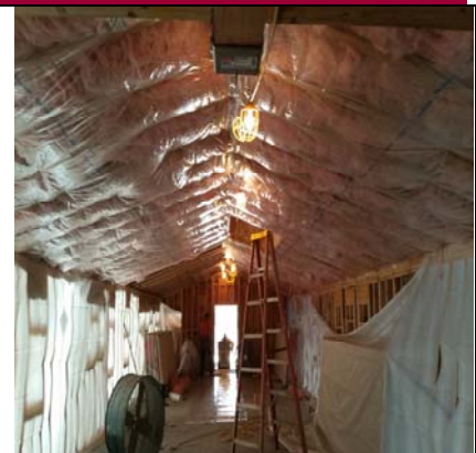
Mechanical Mezzanine Insulation Begins
