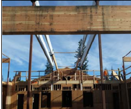
Administration Area Connection Pending
