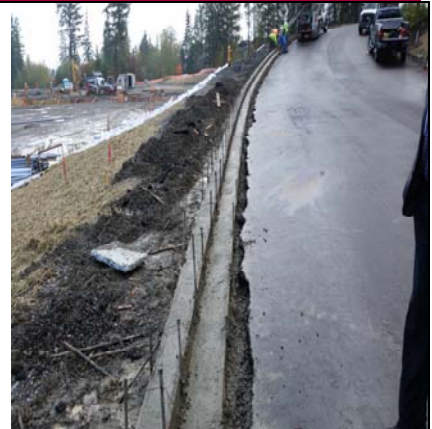
The Cast-In-Place Curbing Begins
