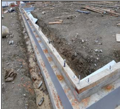
Treated Foundation Top Plates
