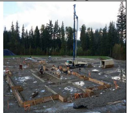
...But Still Ready For Stem Wall Concrete
