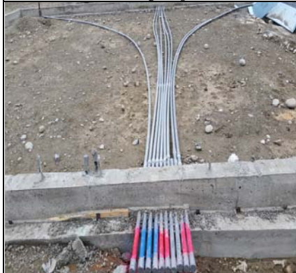
More Under-Slab Electrical & Data
