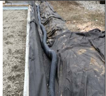
Exterior Footing Drain Installation Begins
