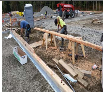
Measuring Up Outside Wall Bottom Plates
