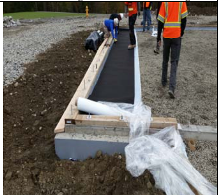
Under-Slab Waterproof Membrane Begins
