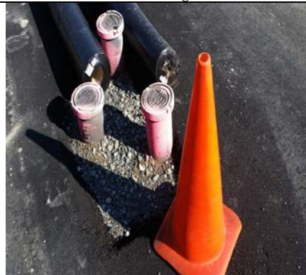
Valve Columns Ready For Final Asphalt
