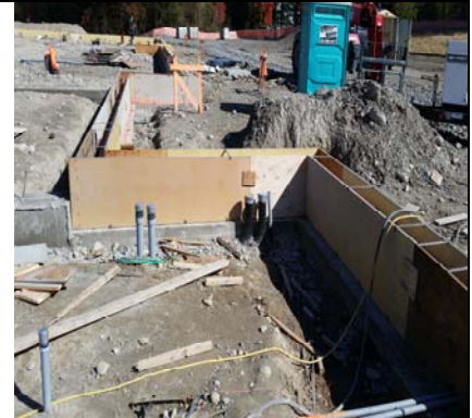
Stem Wall Forms Ready For Concrete
