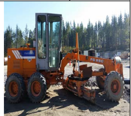
Fine Grading Equipment Ready To Go
