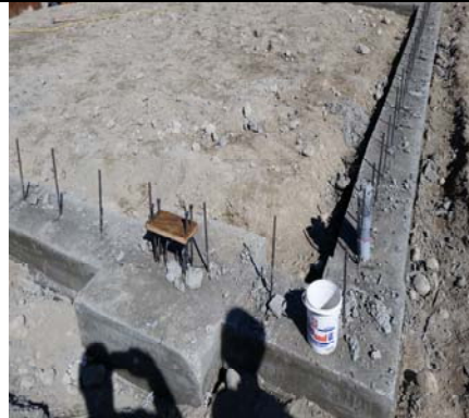
More Footings Ready For Stem Walls
