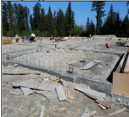
Stripped Footings Ready For Stem Walls
