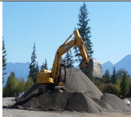
Under-slab Gravel Pending Installation
