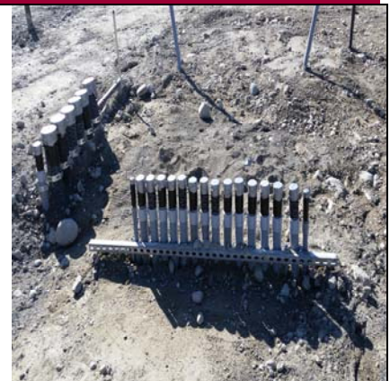
MDF In Ground Main Computer Room
