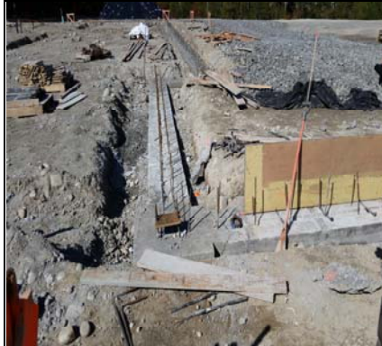
Footings Stripped - Stem Wall Forms Set
