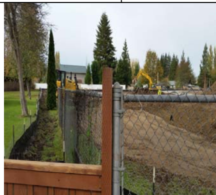
Property Lines Located - Silt Fence Installed
