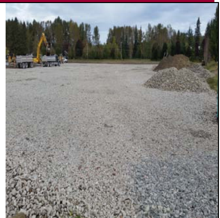
Crushed Rock Construction Pad NE Area
