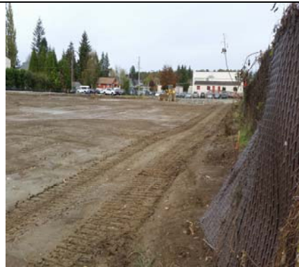
Portable Pad In - Site Rolled For Coming Rains
