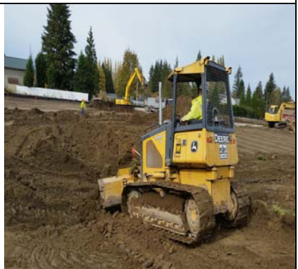
Drainage Ponds Being Dug SE Area
