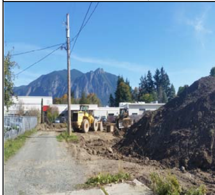
Preparing Pad For Temporary Portables
