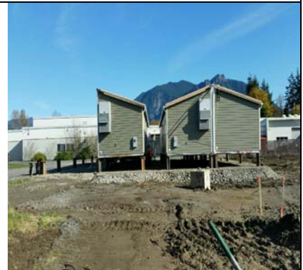
Three Of The Four Halves Arrive On Site
