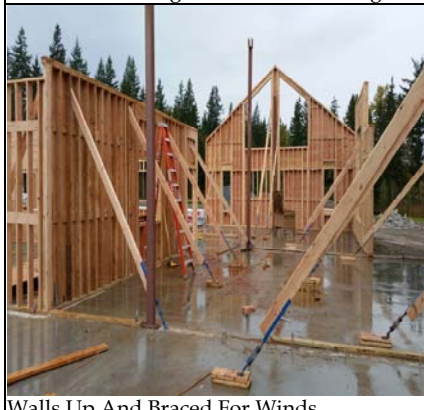
Walls Up And Braced For Winds
