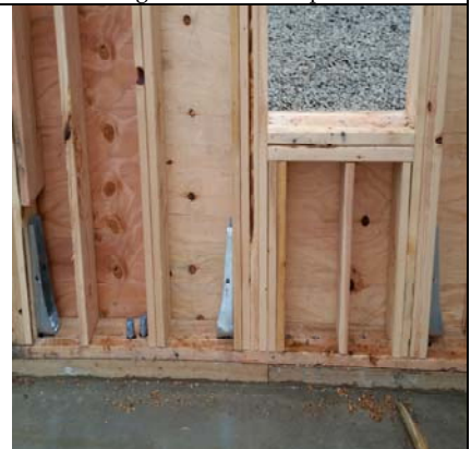
Metal Wall Tie-Downs Everywhere
