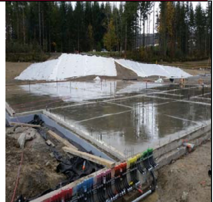
Second Wing Slab Pour Completed
