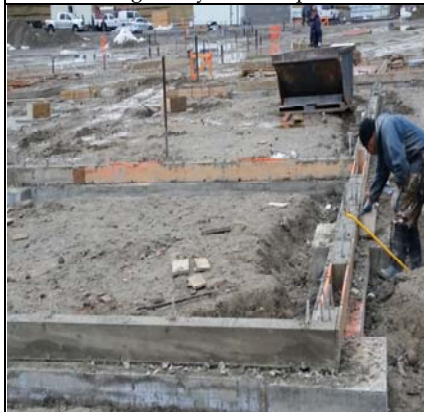
More Forms Being Pulled From Footings
