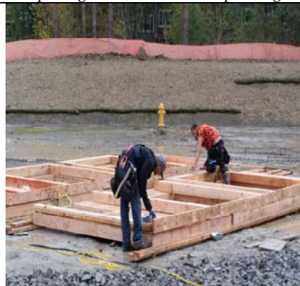
More Exterior Walls Being Constructed
