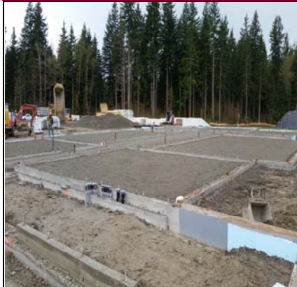
Another Wing Ready For Compaction
