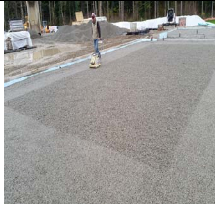
Compacting Rock Prior To Waterproofing
