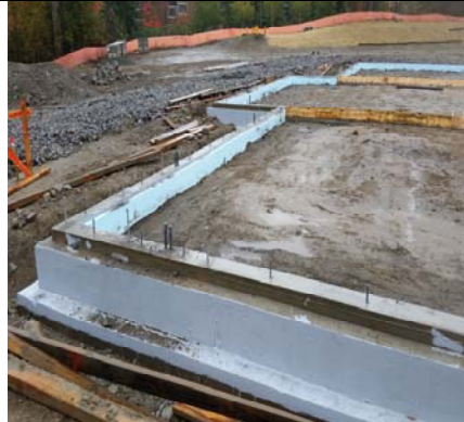
Waterproofing Both Sides Plus Insulation
