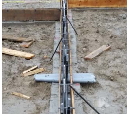
Electrical & Data Feeds To Classrooms
