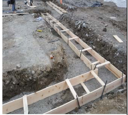
...And More New Footings Being Formed...
