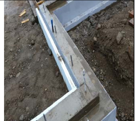
Waterproofing Both Sides Plus Insulation2
