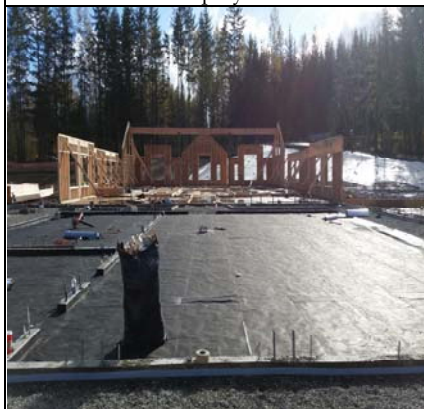
Waterproof Membrane In The Library
