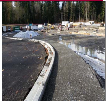
Sub-Base For Sidewalks Begin
