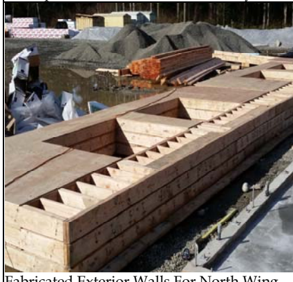
Fabricated Exterior Walls For North Wing
