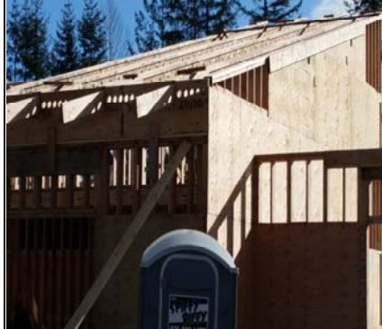
East Wing Rafters - Outside Wall Eaves
