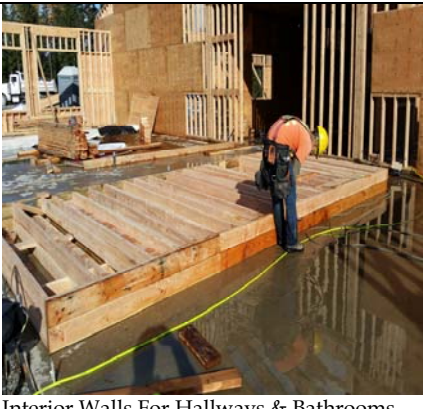
Interior Walls For Hallways & Bathrooms
