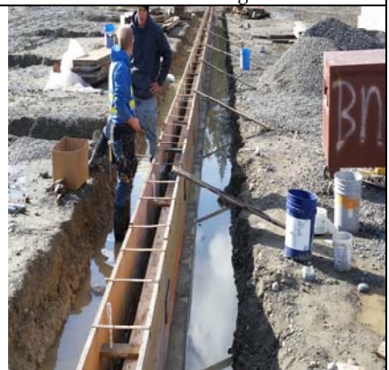
Footings Heading Toward Administration
