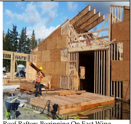
Roof Rafters Beginning On East Wing
