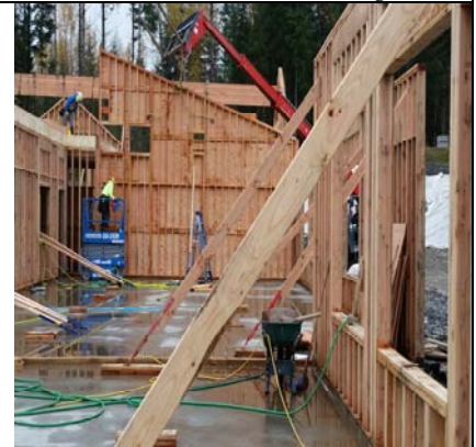
Setting Another Rake Wall
