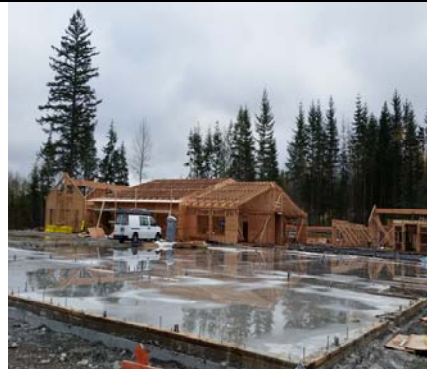
North Wing Ready For Walls
