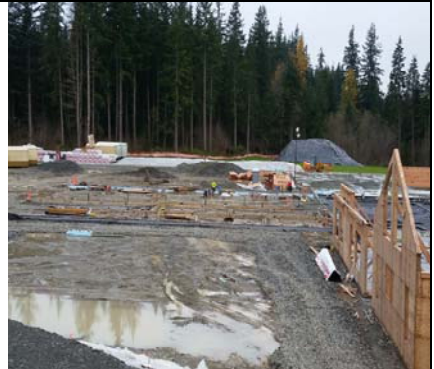
Admin-Area Ready For Water Barrier
