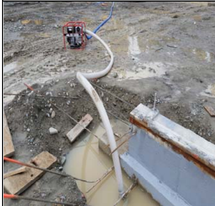
Pumping Water From Every Footing
