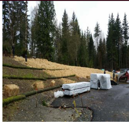
More Straw On All Open Soil Areas
