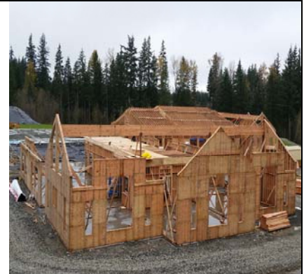
S. Wing Being Readied For Roof Structure
