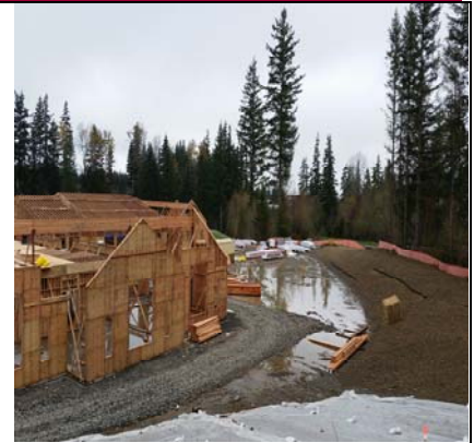
More Rock Road & On Site Holding Pond
