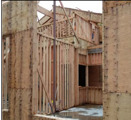
More Interior Walls & Steel Columns
