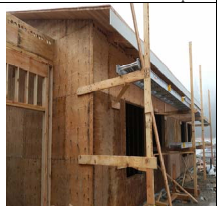
Roof Eaves & Fascia Installations
