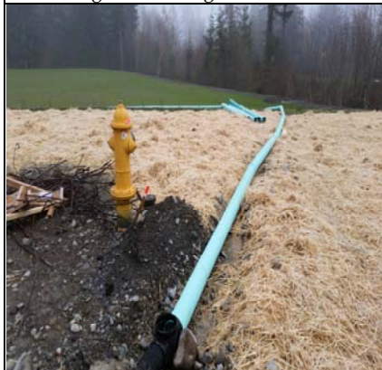
Intercepting The Footing Drains For Now
