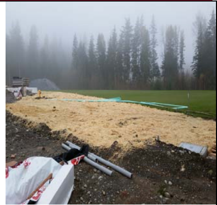
More Straw & Surface Water Flow Pipe
