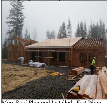
More Roof Plywood Installed - East Wing
