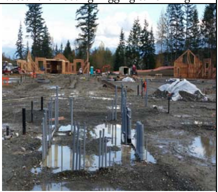
Looking East From The Electrical Room
