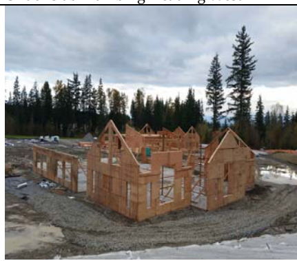
South Classroom Wing Looking Northeast
