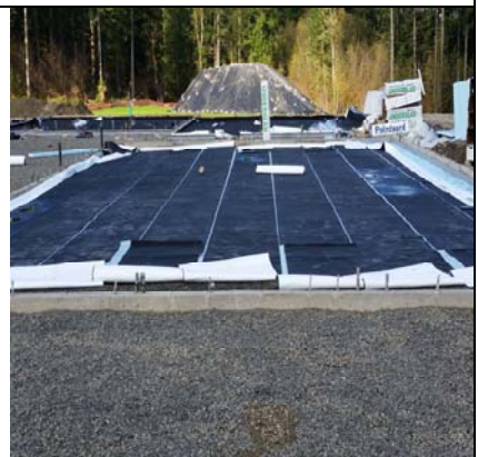
North Wing Water Membrane Installation
