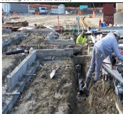
Under-slab Plumbing Heading West
