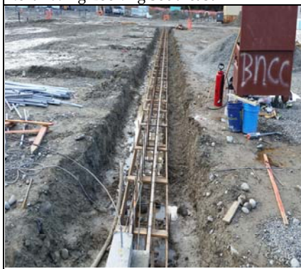
Westward Footing Ready For Concrete
