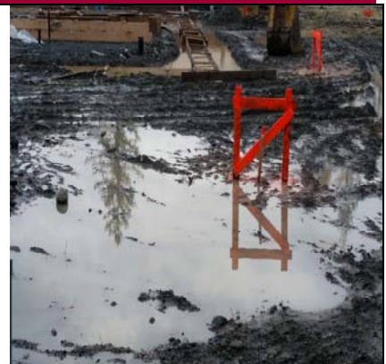
More Footings To Pump Out
