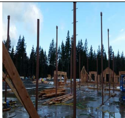
Structural Steel Set In The Library & Core Area
