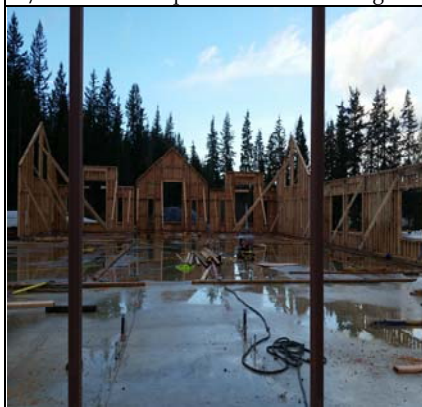
Walls Going Up In The North Wing
