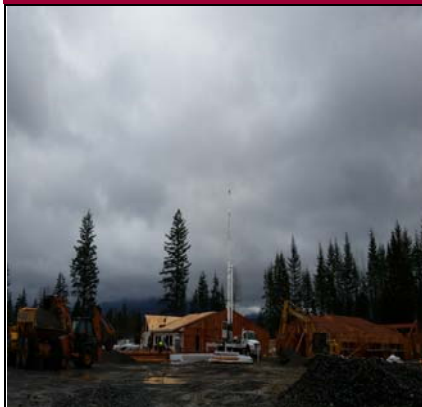
12/8 - Crane Setup - More Rain Coming
