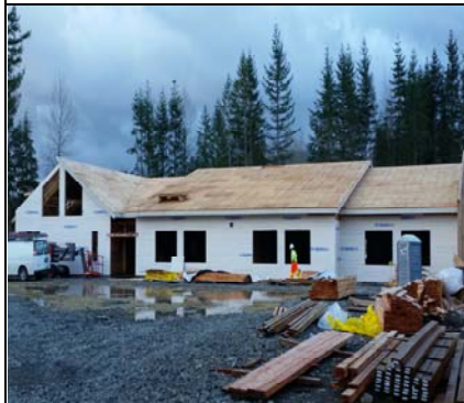
Weatherboard Over Sheathing East Wing
