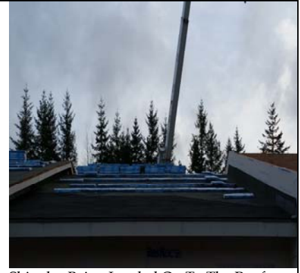
Shingles Being Loaded On To The Roof
