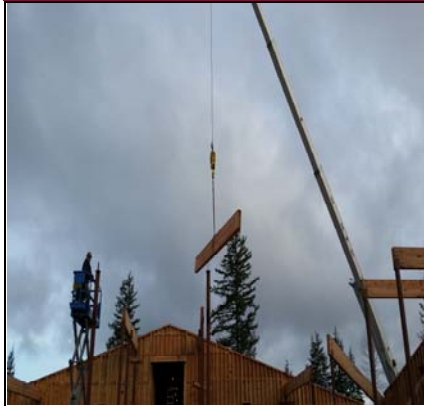
Setting Library & Core Beams
