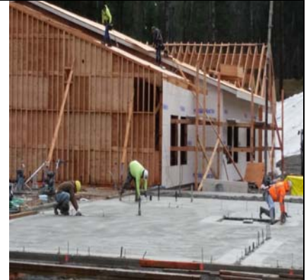
Hand Finishing Concrete Slab
