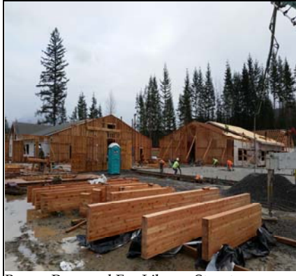
Beams Prepared For Library Structure
