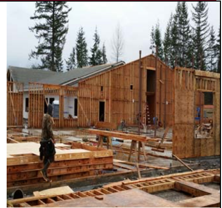
North Wing Walls By Library
