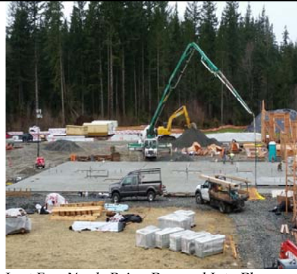
Last Few Yards Being Pumped Into Place
