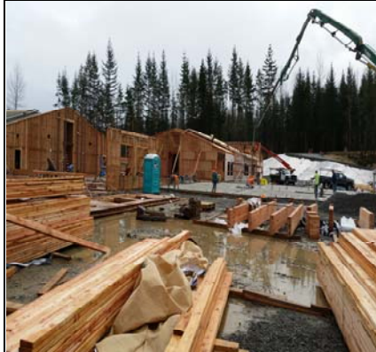
12,000 Square Foot Slab Pour-Admin Area
