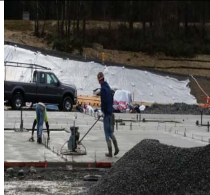
Power Finishing Concrete Slab
