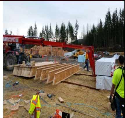
More Truss Preparation - More Trusses
