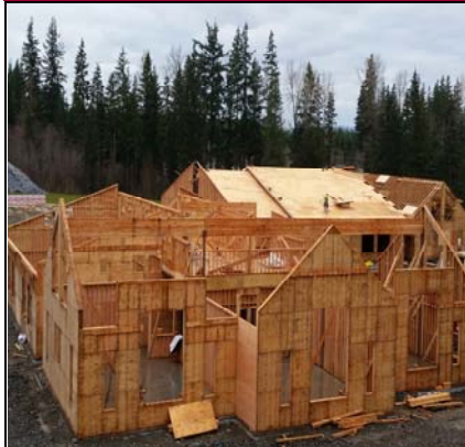
More Roof Sheathing - Mechanical Space
