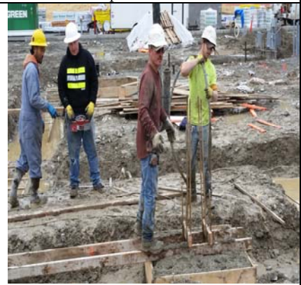
Entry Column Footings/Foundations 2
