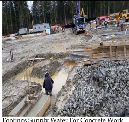
Footings Supply Water For Concrete Work
