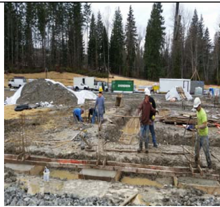
Entry Column Footings/Foundations
