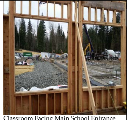
Classroom Facing Main School Entrance
