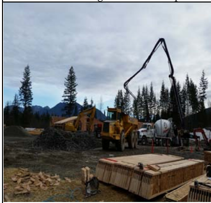
More Concrete Footings & Foundations
