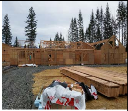
Trusses Heading For Walls
