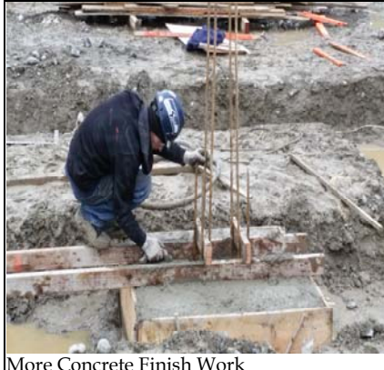
More Concrete Finish Work
