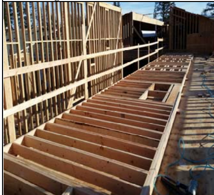
Administration - HVAC Mezzanine Walls
