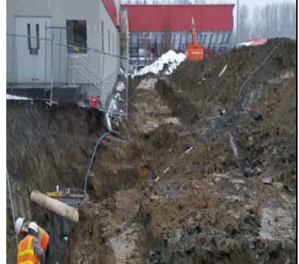
Preparing For Temp Retaining Wall At Bldg
