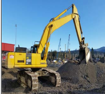
Subgrade Haul Out - Cranes Advancing
