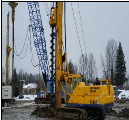
Drilling Pilot Hole For Lg-Crane Probe
