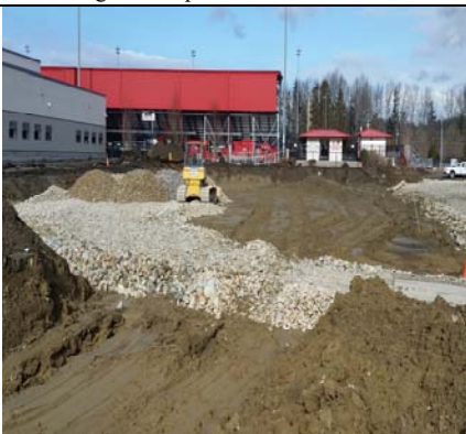
Subgrade Achieved/Rock Pad Installation
