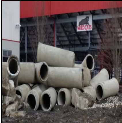
Pre-Existing Storm Drainage Removed
