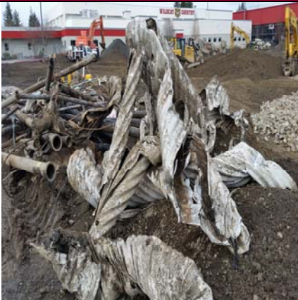
An Assortment Of Underground Removals
