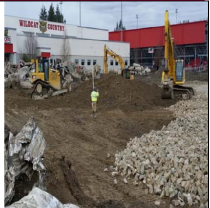
Sidewalk Haul Out - Getting To Subgrade
