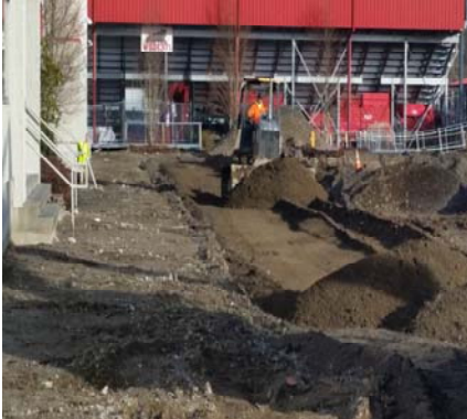
More Subgrade Preparation For Haul Out
