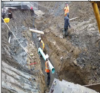
Manhole Installations/Sewer Relocations
