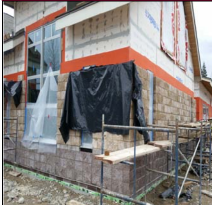
East Wing Exterior Masonry - North Side
