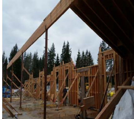
Kindergarten North Walls & Center Beam
