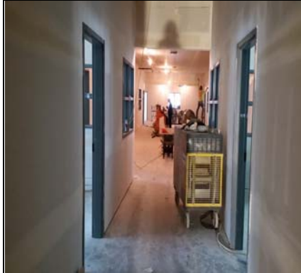
East Wing - Hallway - Temp-Heat On
