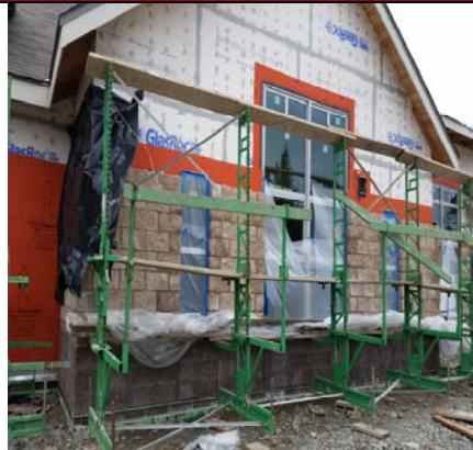
East Wing Exterior Masonry - East End
