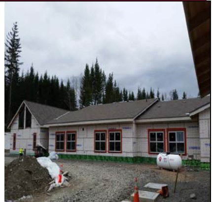
South Wing - Being Prepared For Masonry
