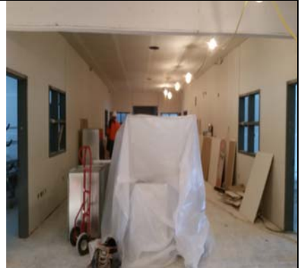
South Wing - Hallway - Sheetrock
