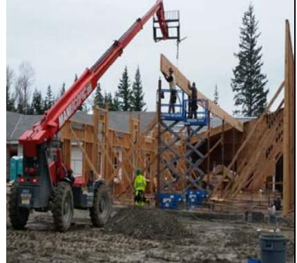
Last Kindergarten Beam Being Set
