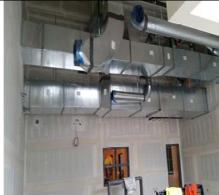
South Wing - Sheetrock - HVAC Ductwork
