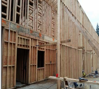
Kindergarten Hallway - N Side South Wall
