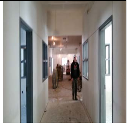
East Wing - Primed/Prepared For Paint
