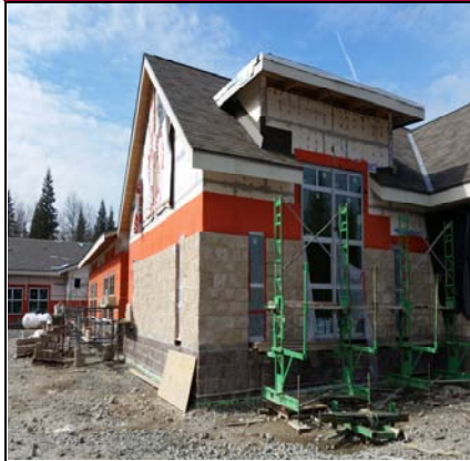
East Wing Exterior Masonry - South Side
