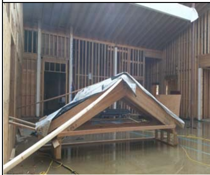
Remaining Clerestory Beams Constructed
