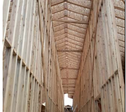
Library Hallway - Clerestory Opening
