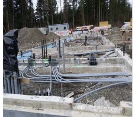
Electrical Room-Kitchen-Gym Bathrooms
