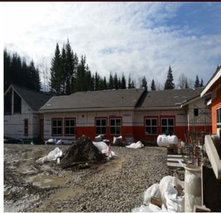
South Wing Exterior Masonry - East Side
