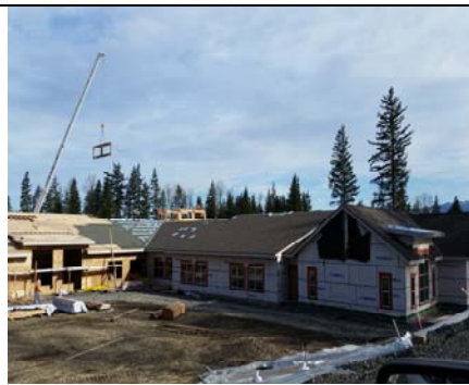
2/26 Crane Set - Clerestory Construction -1
