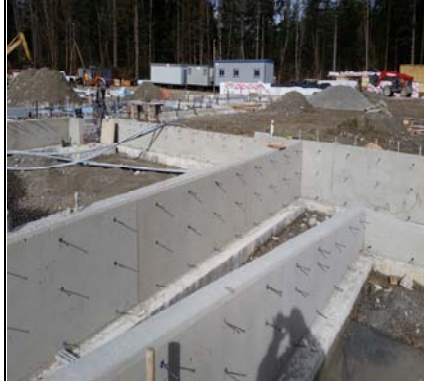
Ramp Walls For Stage Ramp Access
