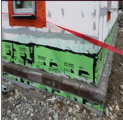
Air/Water Barrier Bottom Seal -Base Block
