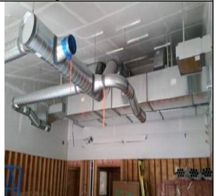
...Next Room Sheetrock - Ductwork
