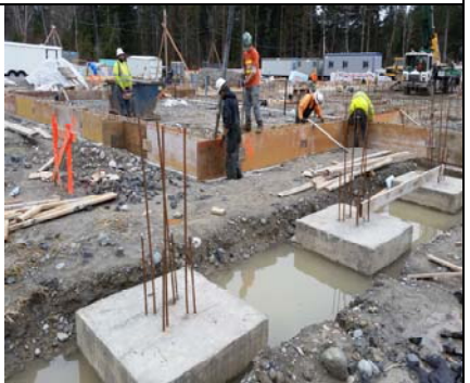
Pouring West Wing/Stage Stem Walls
