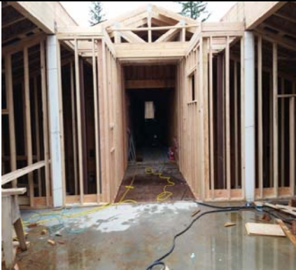
Final Mechanical Mezzanine Connections
