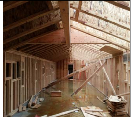
North Wing Mezzanine Final Enclosure
