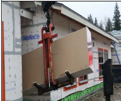
Loading More Sheetrock Into The Building
