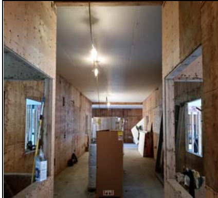
Hallway Ceiling Sheetrock Installed
