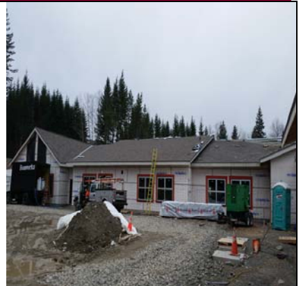
South Wing Windows/Roof - Dried-In
