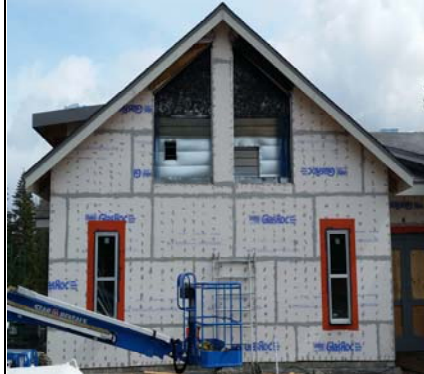
Large Air Ductwork Ready For Louvers
