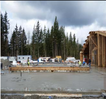
Northwest Wing/South Ready For Walls
