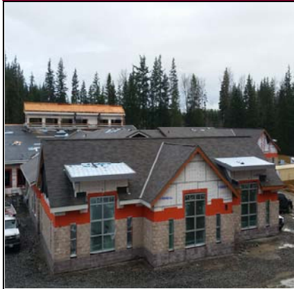
South Wing - Ready For Capstone/Siding
