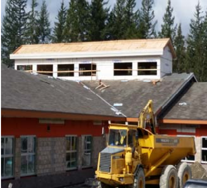
S-Wing Ready For Gutters & Downspouts
