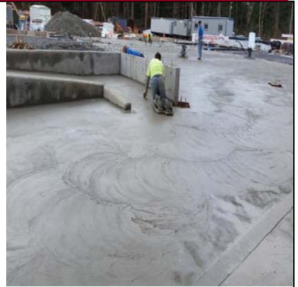
Concrete Finish Of Hallways & Ramps
