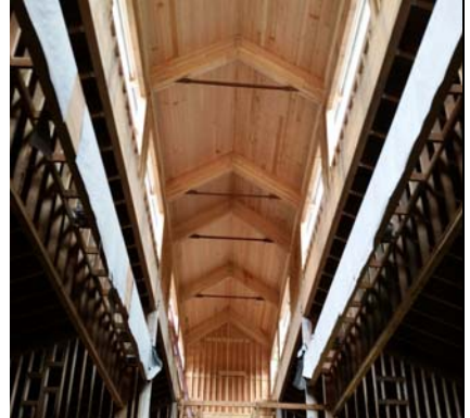
Clearstory - Ready For Deco-Crossbeams
