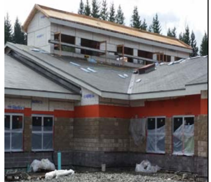
North & East Wing Tie-In & Clearstory
