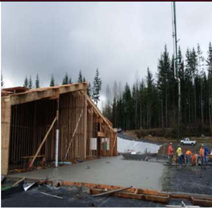
Concrete Pour In Multi-Purpose Area
