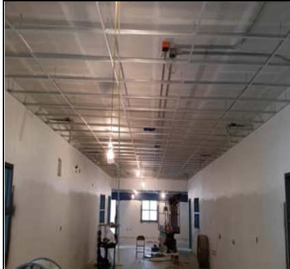
East Wing Ceiling Grid - Casework Next
