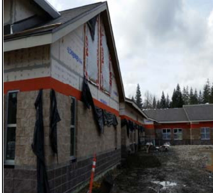
East Wing Ready For Capstone & Siding
