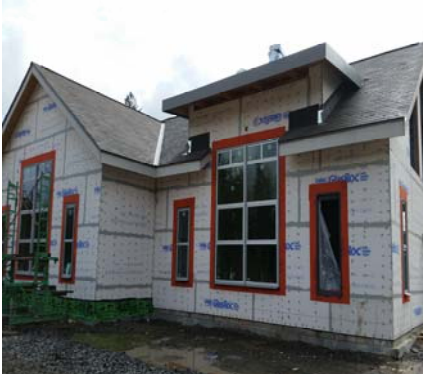
North Wing Ready For Membrane & Block
