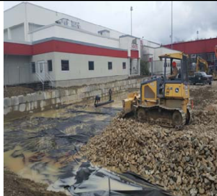
Moving In The Spall Rock Pad
