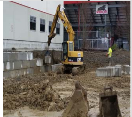
Finishing The Temporary Retaining Wall
