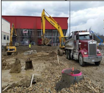
...Finally The Last Soil Haul Out
