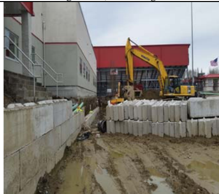
Final Material For Temporary Retaining Wall
