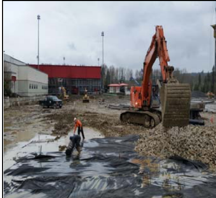
Adding Geo-Fabric For Extra Pad Stability
