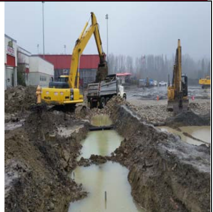
More Holding Ponds/Moving Out Soil
