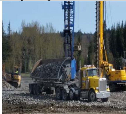
Additional Rock For Pad Stability 2
