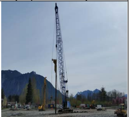
Large Crane Left To Finish Stone Columns
