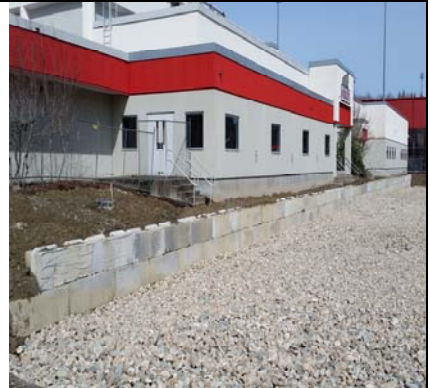
Temporary Wall & Pad Complete & SUN
