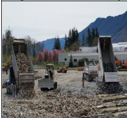
Additional Rock For Pad Stability 1
