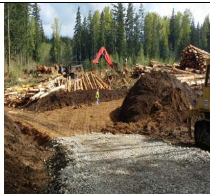
Site Facing Easterly 1 - Haul Road Exit
