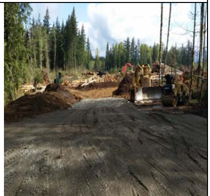
Site Facing Easterly 2 - Haul Road Exit
