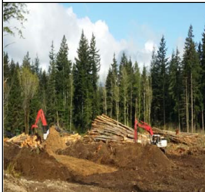
Site Facing Northwesterly
