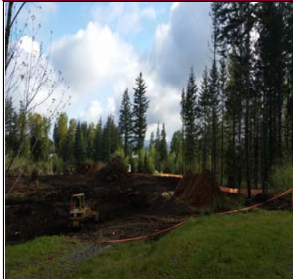
Site View Facing Northeast
