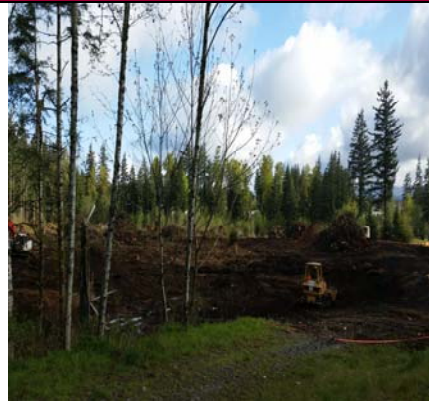
Site Facing North
