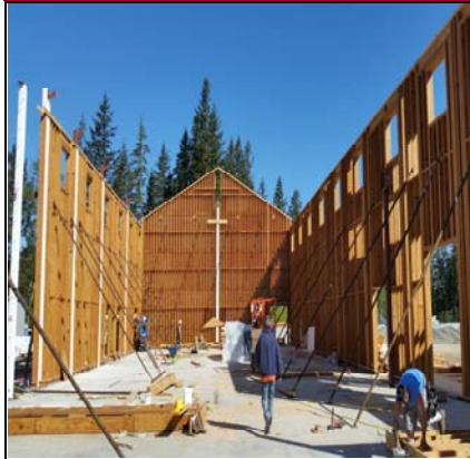
NW Wing - Gym Walls Looking North
