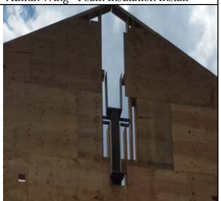
Steel Column Awaiting 100' Gym Beam...
