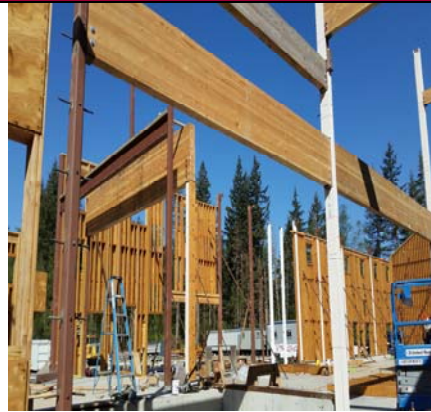
NW Wing - Stage & Hallway Beams
