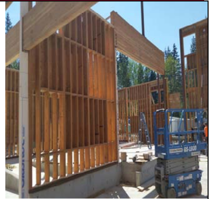
NW Wing - Stage Walls
