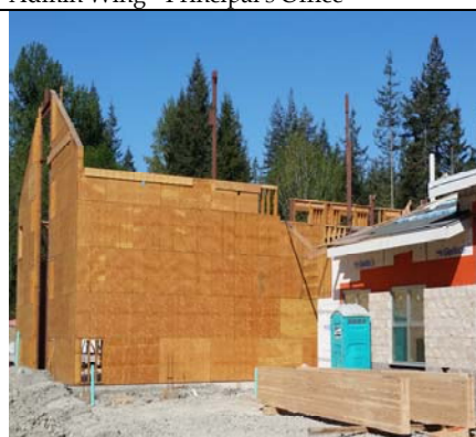
Entryway Beams Prepared For Install
