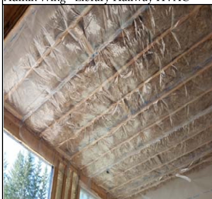
Admin Wing - Insulation Install
