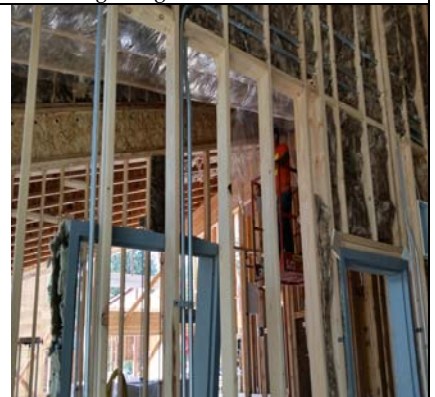
Admin Wing - Hollow Metal Door Install
