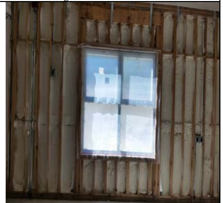
Admin Wing - Foam Insulation Install
