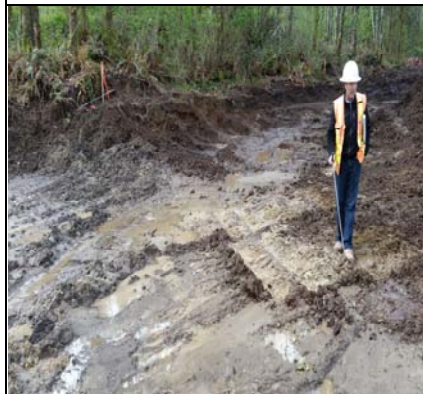
Soil Stability Inspection
