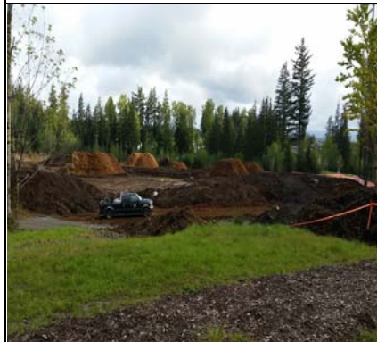
Site View Northeast
