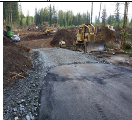
Haul Road Construction
