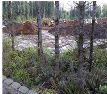
Site View Northeast 2
