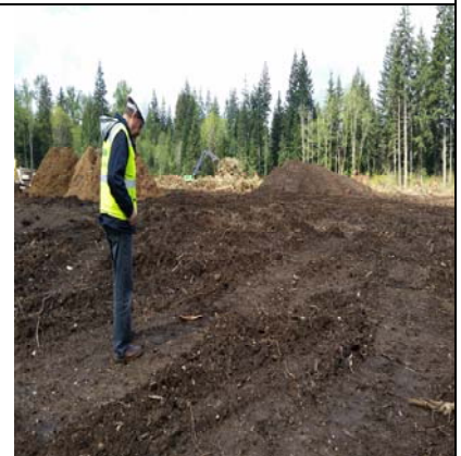
Site Clearing Inspection
