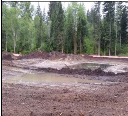
Protective Holding Ponds
