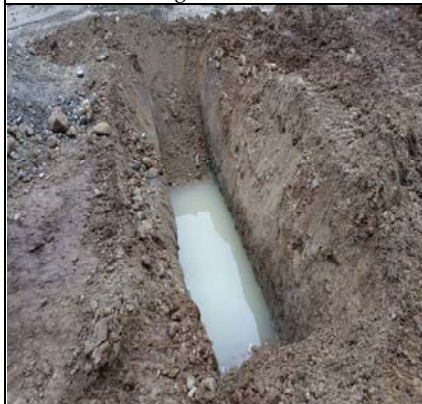
One of Two Test Pits - Perched Water
