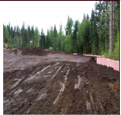
Site View West 2 - Soil Too Wet To Work
