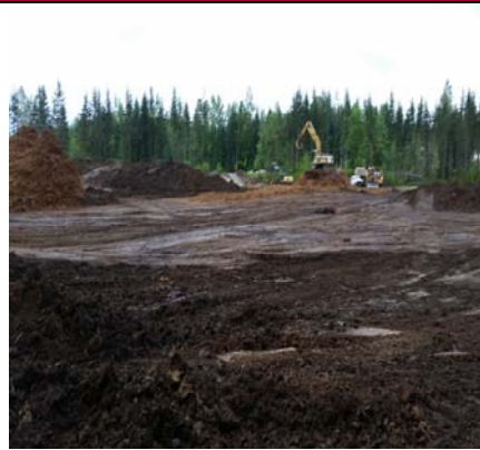
Site View West - Compacted For Protection
