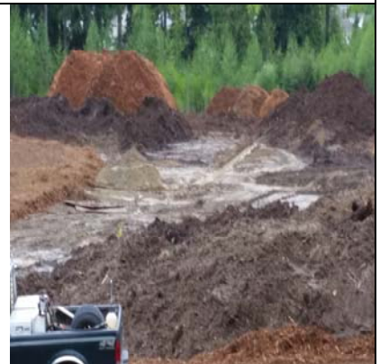
Site View North - Too Wet To Work
