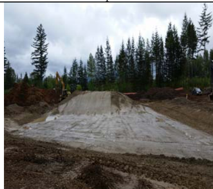
Site View East - Compacted For Protection
