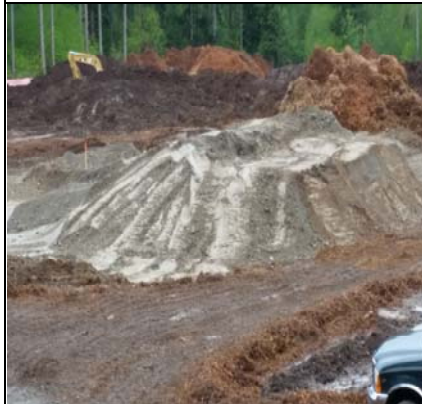
Site View North - Too Wet To Work
