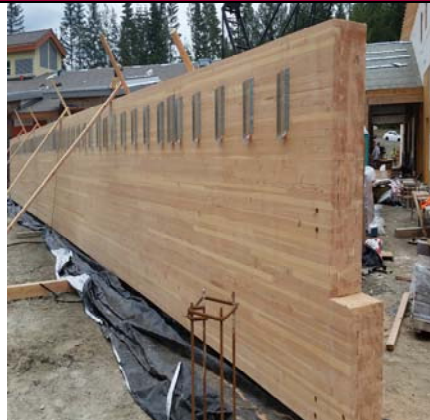
Gymnasium Beam Prepared For Install
