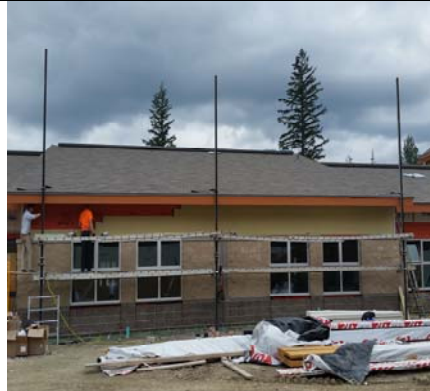
Lower Level Siding Has Begun
