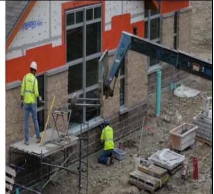
Precast Capstone/Sill Installation Begins
