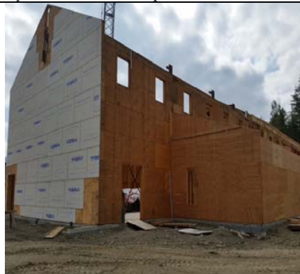
...Pending Beam Installation-Trusses To Follow
