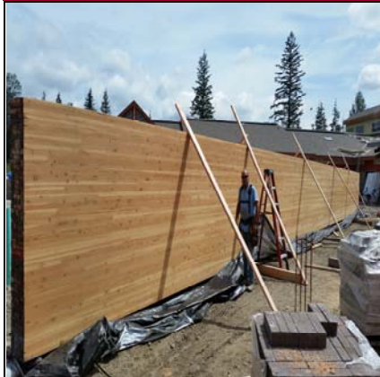
100' Gymnasium Beam Arrival
