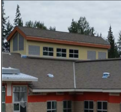
Clearstory Siding Complete
