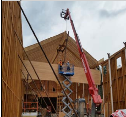
Setting Structural Steel Beam Connector
