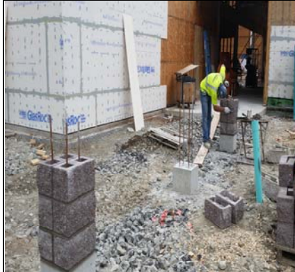
Entryway Column Masonry Has Begun
