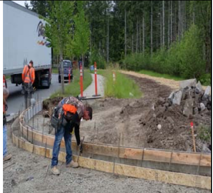
Main Entry Road Connection Has Begun
