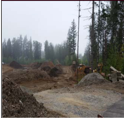
Site View Northeast - 5/20
