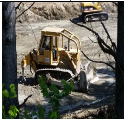
Southwest Site Corner - Subgrade - 5/21
