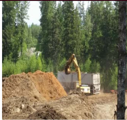
Site View Northeast 2 - 5/21 Chip Hauling
