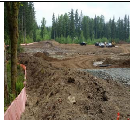
Site View From Northwest Corner - 5/20
