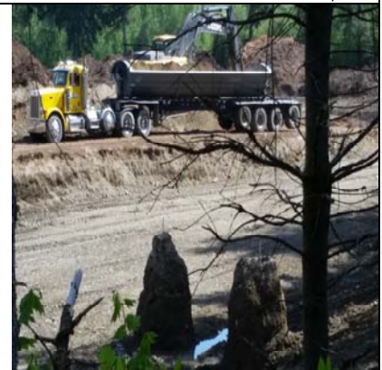
Site View Northeast 3 - 5/21
