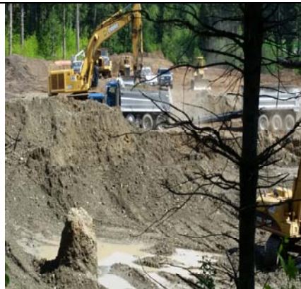
Site View Northeast 2 - 5/21
