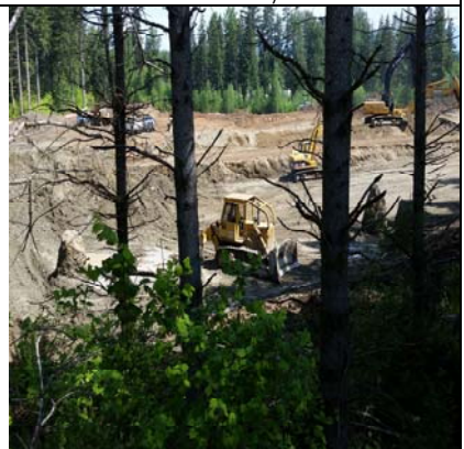
Site View Northeast 4 - 5/21
