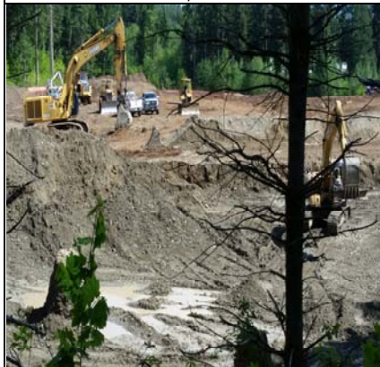
Site View Northeast - 5/21
