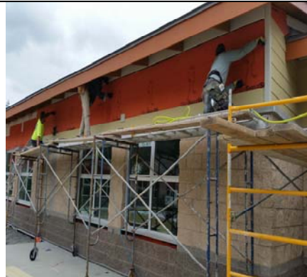
Siding Installation Chasing Masonry
