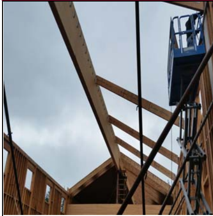
100' Gymnasium Beam Set In Place
