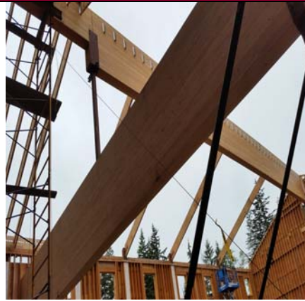
Gymnasium Roof Beam Connections
