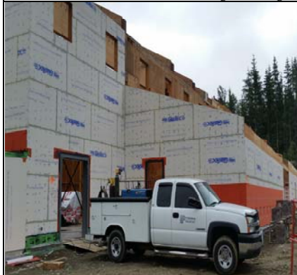
Ready For Masonry West Wall - NW Wing
