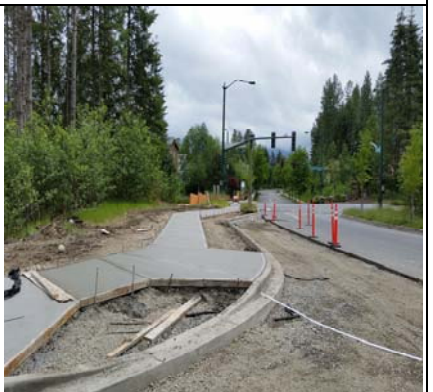
Main Entry Sidewalk - East Side
