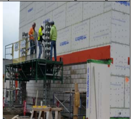
Masonry At North Wall - NW Wing
