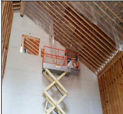
Insulation & Sheetrock Following Roofing
