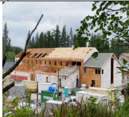
NW Wing View From Southeast
