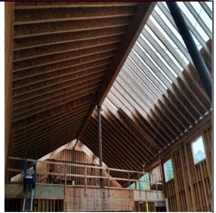
Gym Trusses & Sheathing Following
