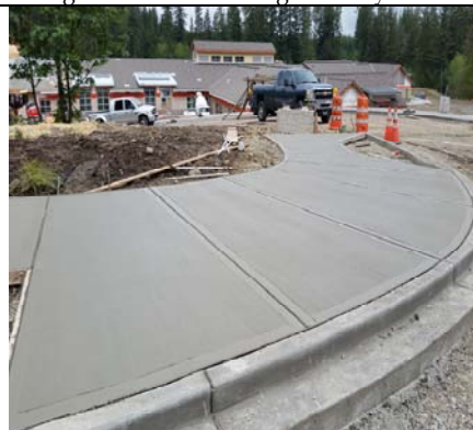
Main Entry Sidewalk - West Side
