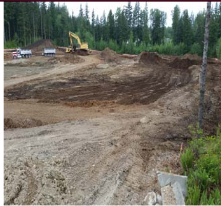
Site View Northeast 2
