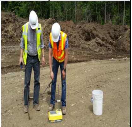
Moisture & Compaction Testing
