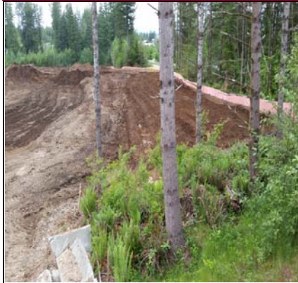
Site View Northeast
