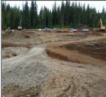
Site View North
