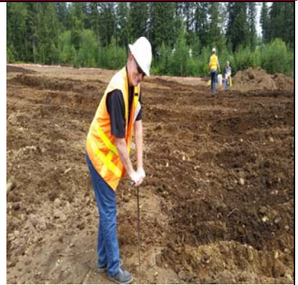
Sub-Grade Soil Testing
