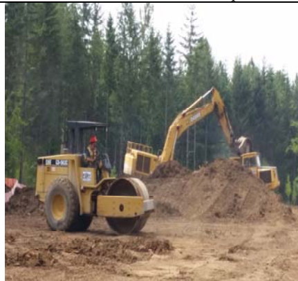
Subgrade Compaction Begins
