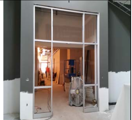
Library Windows & Doors Going In
