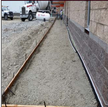
Sidewalk Compacted Ready For Concrete
