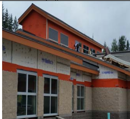
Clearstory Weather Sealed - Siding Begins
