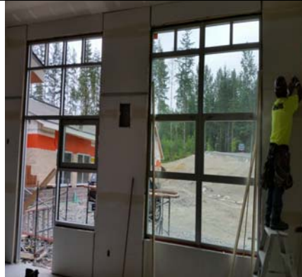
Sheetrock & Taping Inside Storefronts
