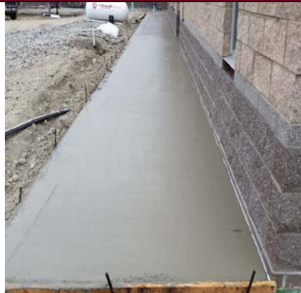
Concrete Sidewalks Begin
