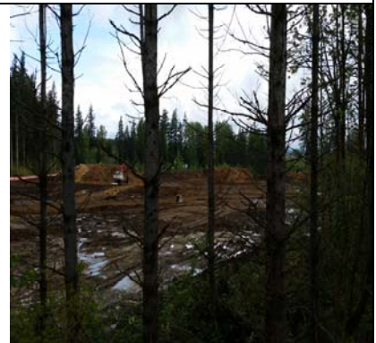
Site View Northeast
