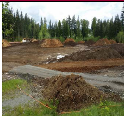
Site View North
