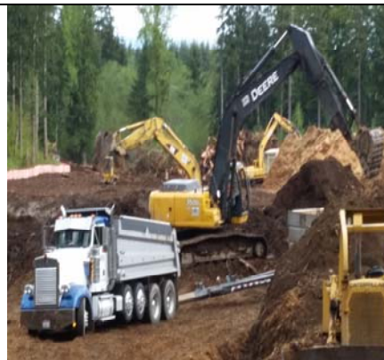
Truck Topsoil Loading 3
