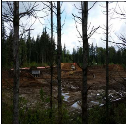
Site View Northeast 2
