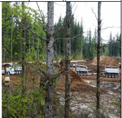
Multiple Truck Topsoil Haul Operation
