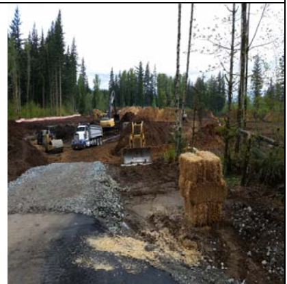
Truck Topsoil Loading
