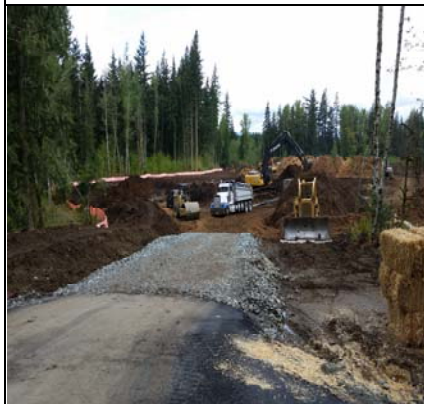
Truck Topsoil Loading 2
