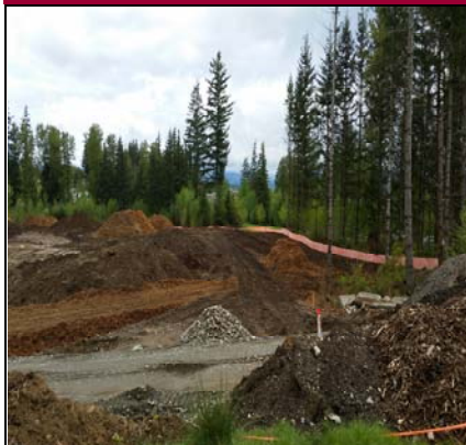
Site View Northeast
