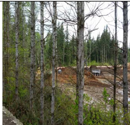
Site View Northeast 3
