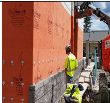
NW Wing - Masonry Block Continues
