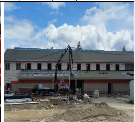
NW Wing - Roofing Nearing Completion
