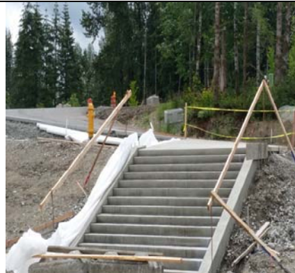
Grand Entry Staircase
