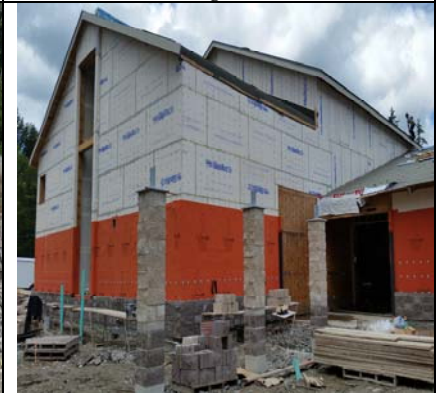
Entry - Weatherproofing Continues
