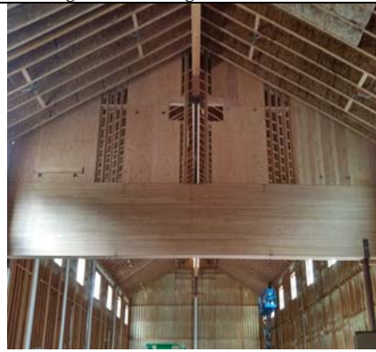
Multi-Purpose/Gym Operable Wall Opening
