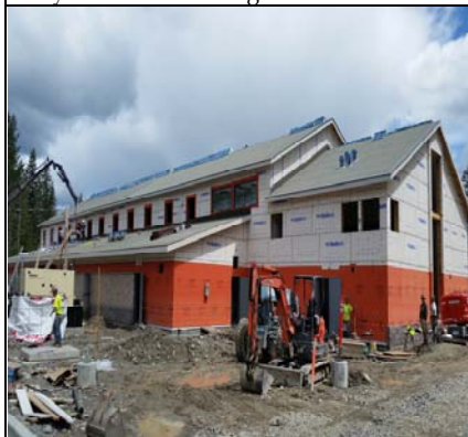
NW Wing - Weather Proofing Continues
