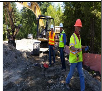
Backfilling & Compaction Testing
