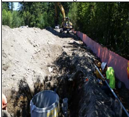
Setting A Base Structure 2
