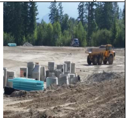
Moving Soil Across The Pad To The Field
