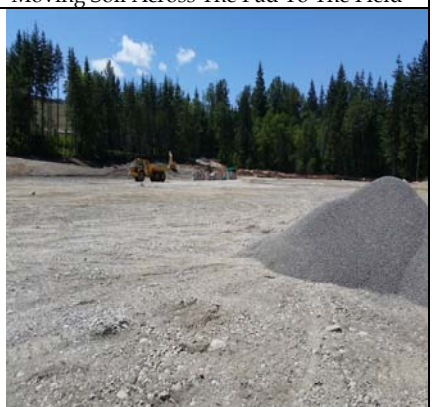
Site View - S.W. Across The Building Pad
