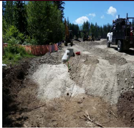
Sanitary Sewer Installation Has Begun
