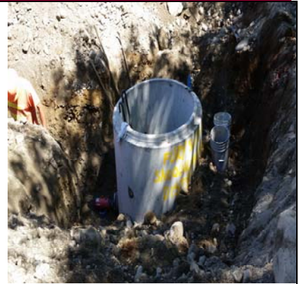
Setting A Base Structure
