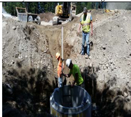
Laser Leveling To The Next Structure
