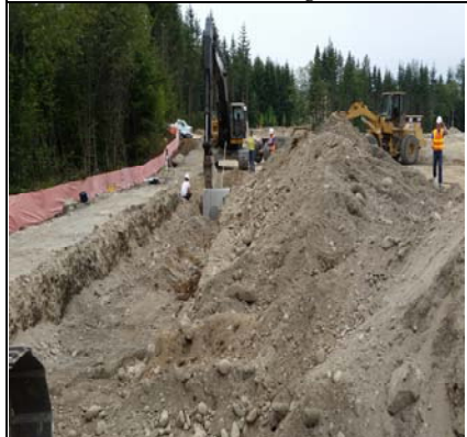
Storm Drainage Backfill
