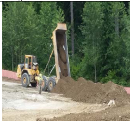
Continuing To Spread The Stockpile
