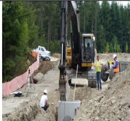
Setting Another Manhole
