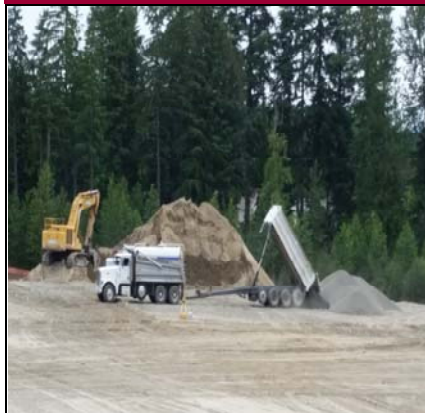
Stockpiled Soil & Pipe Bedding Delivery
