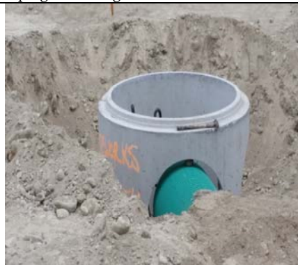
Initial Storm Drainage Structure
