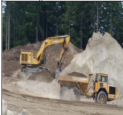
Continuing To Haul The Stockpile
