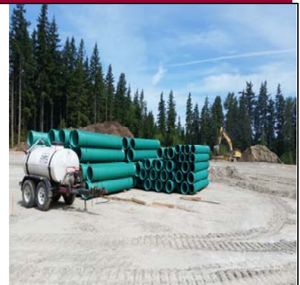
More Drainage Piping
