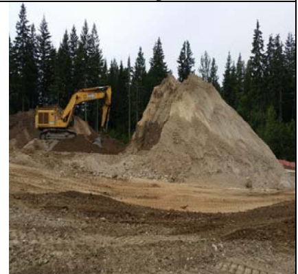
Continuing To Process The Stockpile
