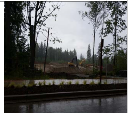
Rain/Not Going To Be OK - 6/2 & 6/3
