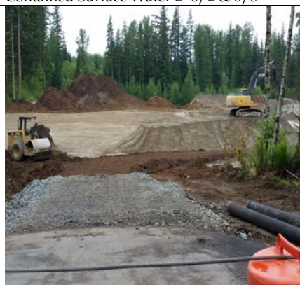
Site Left In Compacted State - 6/2 & 6/3
