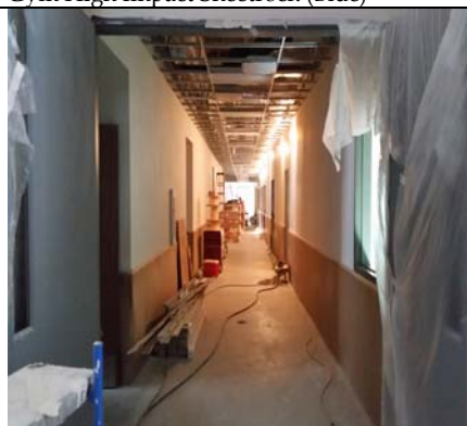
Main Hallway Pending Flooring & Ceiling
