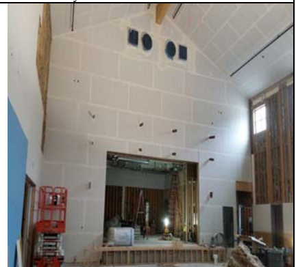
Multi-Purpose Area/Stage Sheetrock
