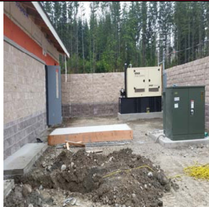
Main Power-Generator-Gas Line Install
