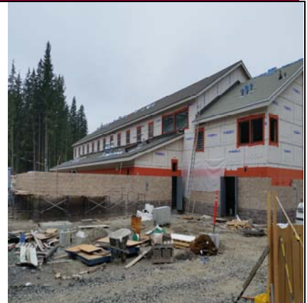
NW Wing With Utility Area Walls
