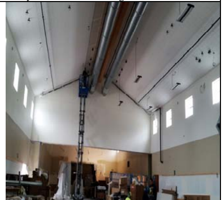
Gym & Multi-Purpose Trimming Out
