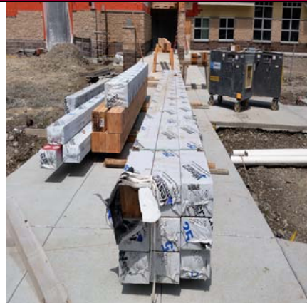
Entry Structure Package Arrival
