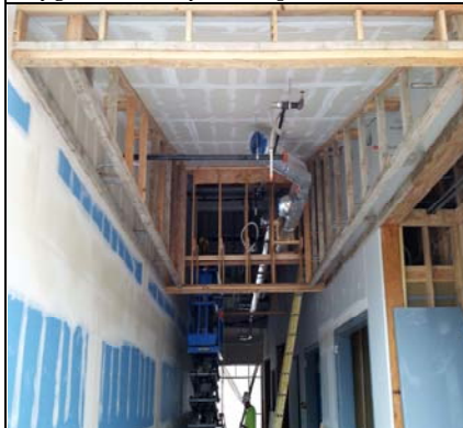
Entry Soffits Being Framed
