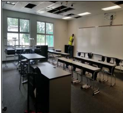
Classrooms Being Trimmed Out
