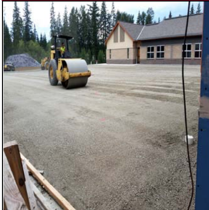
Playground Ready For Asphalt
