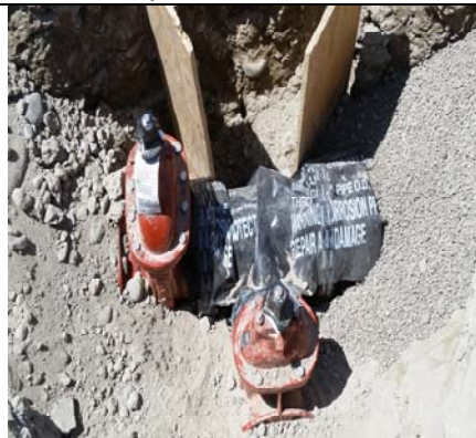
Valves Ready For Concrete Thrust Blocks
