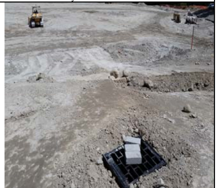
Building Subgrade And Drainage
