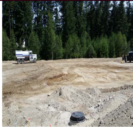
More Playfield Area & Utility Berm
