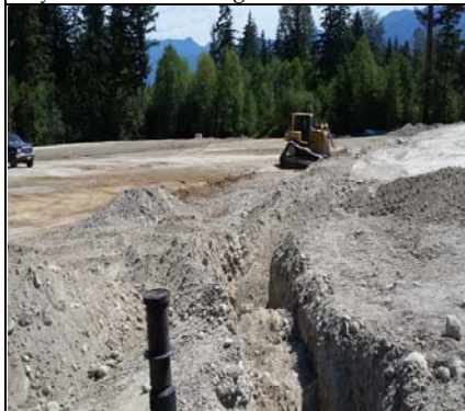
Water Main Coming By The Playfield
