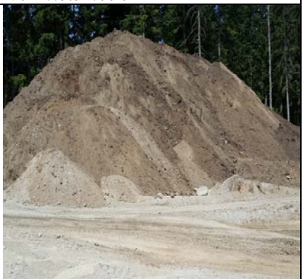
Topsoil Stockpile Pending Processing
