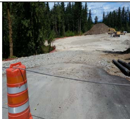
Bus Loop To Subgrade
