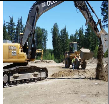
More Trenching For Drainage Pipe
