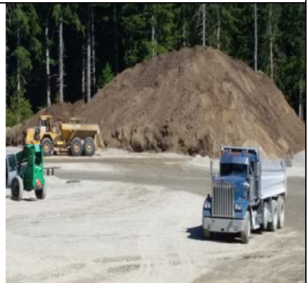
Topsoil Stockpile Pending Processing
