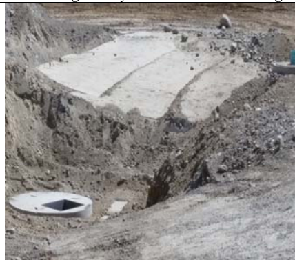
Drainage Near The Field
