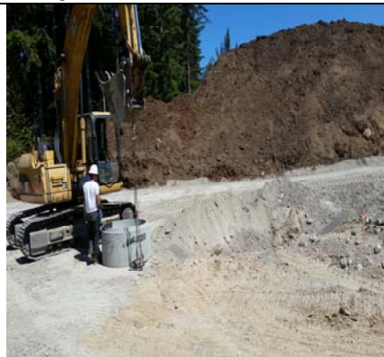
Setting Another Manhole
