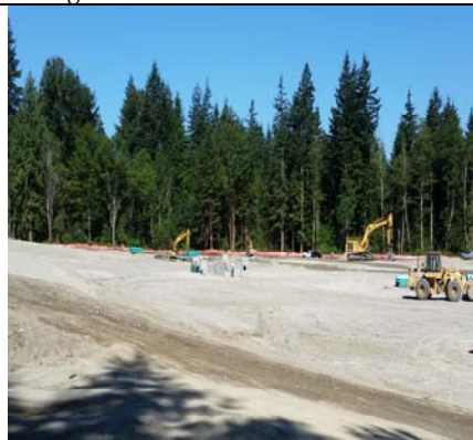
Site Entry Looking Northwest
