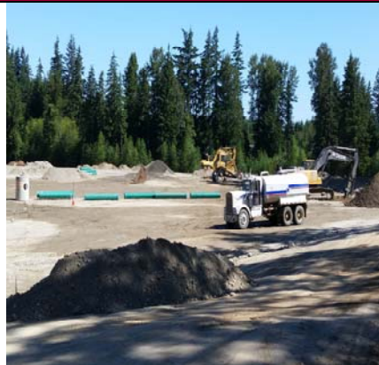
Continuing To Lay-out The Storm Drainage
