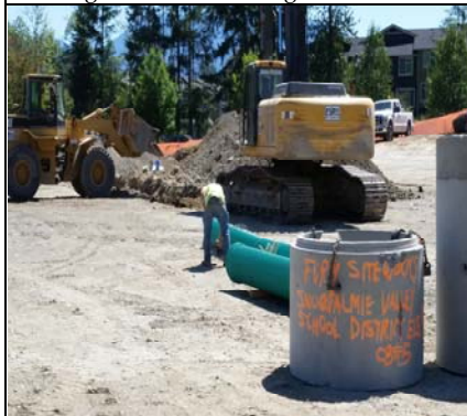
Installing Drainage Pipe
