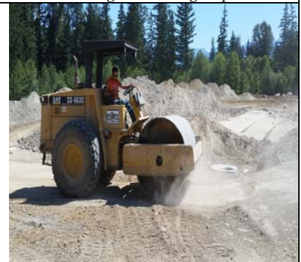
Another Lift Of Field Soil Compaction
