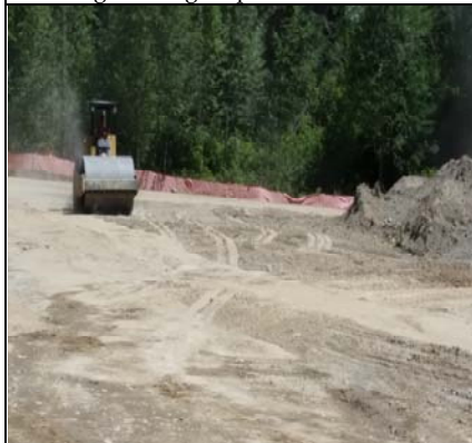
Another Lift Of Field Soil Compaction 2
