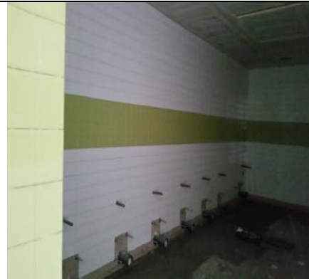
Gym Restrooms Awaiting Grout & Fixtures
