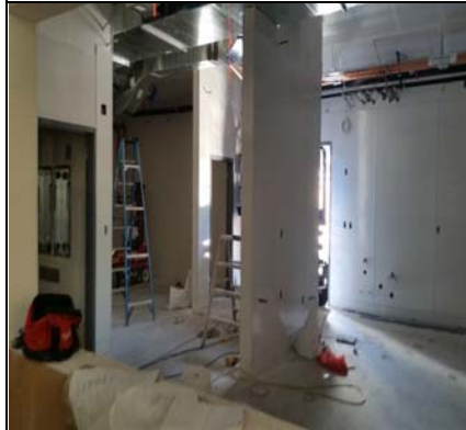
Kitchen Awaiting Walk-in Freezer/Cooler
