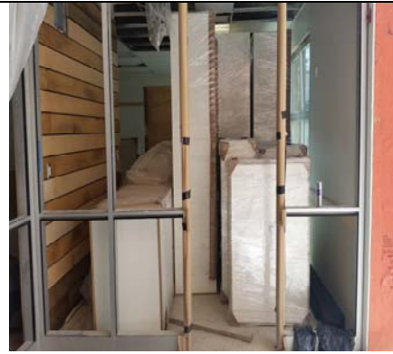
Admin Entry Storing More Casework
