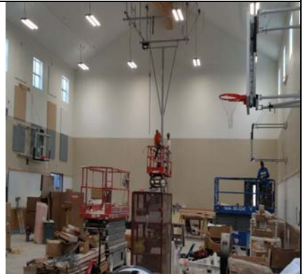
Gym Acoustical Tile - Lights - BB Hoops
