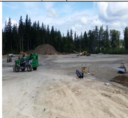
Nearing Pad Ready - Topsoil Processing
