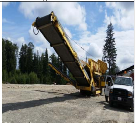
Topsoil Processor Set-Up
