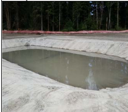
Temporary Sediment Pond/Water Test
