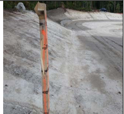
Storm Drainage Stubs - Trench Drain
