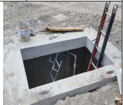
Water Main Vault
