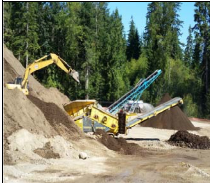
Sorting The Rocks & Debris From Soil
