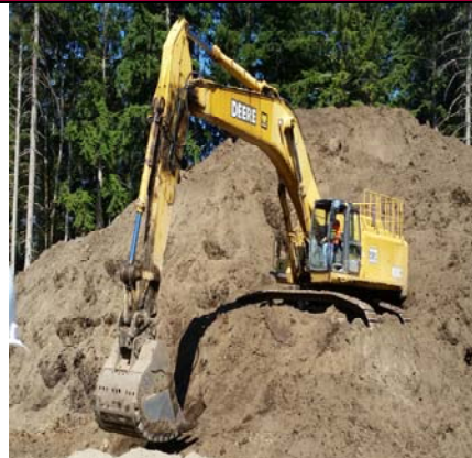
Making The Stockpile Smaller
