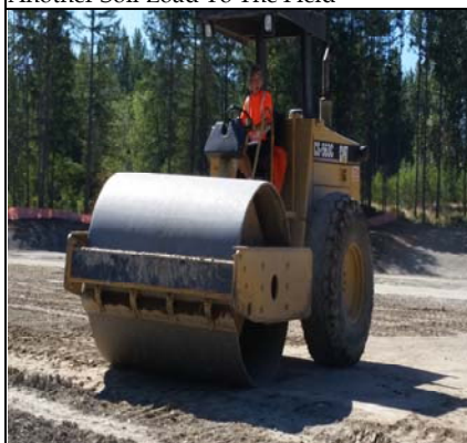
Another Soil Lift Being Compacted
