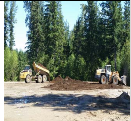
Another Soil Lift Being Spread
