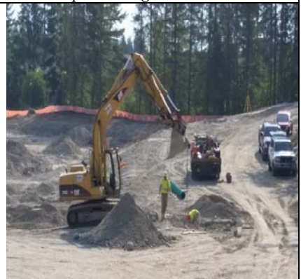
Working On The Storm System
