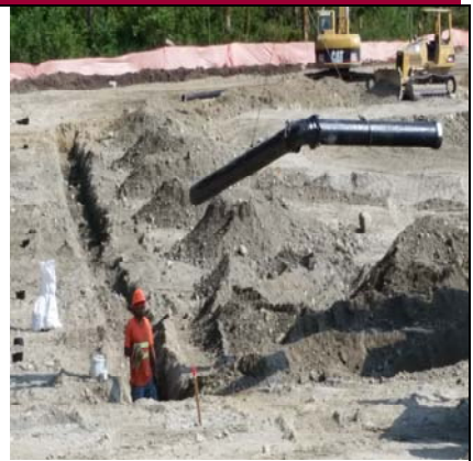
Installing The Water Mains
