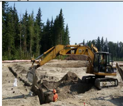
Backfilling The Water Main - Turn The Corner
