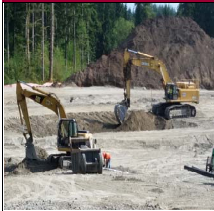
Digging The Temporary Sediment Pond
