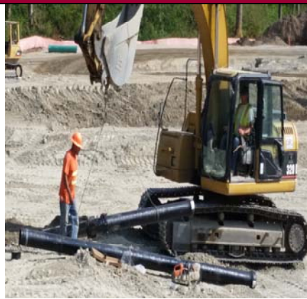
Setting Up To Install Water Mains
