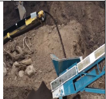
Transferring Up To New Soil Stockpile
