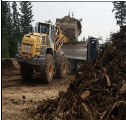
Loading The Spoils Out & Off-Site
