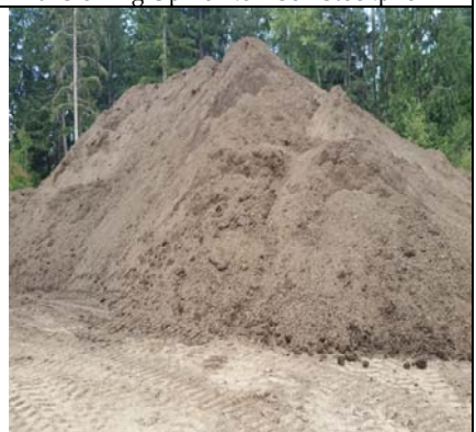
Building A Stockpile For Phase 2
