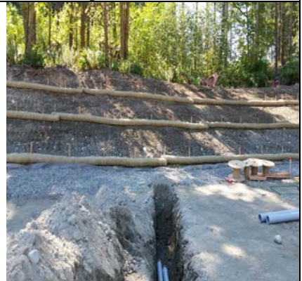
Main Electrical Feed To The Building 2
