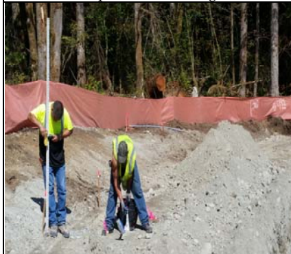
Staking Out The Parking Lots For Rock
