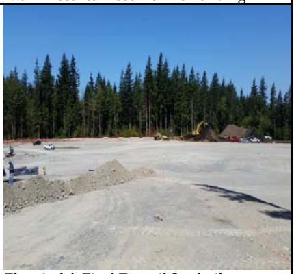
Electrical & Final Topsoil Stockpile
