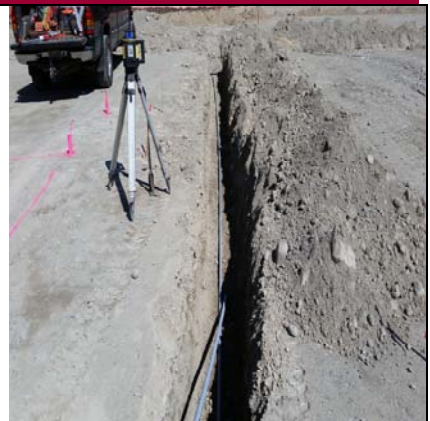
Laser Set - Underground Electrical
