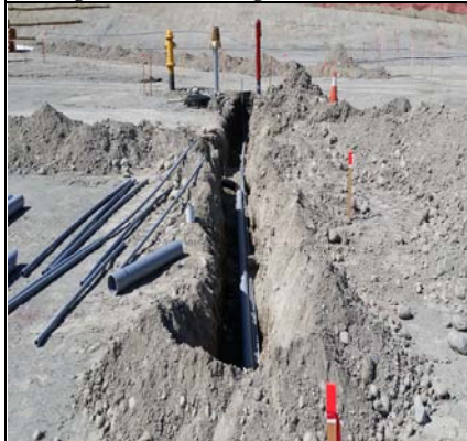
More Underground Electrical
