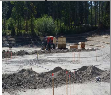
More Underground Electrical
