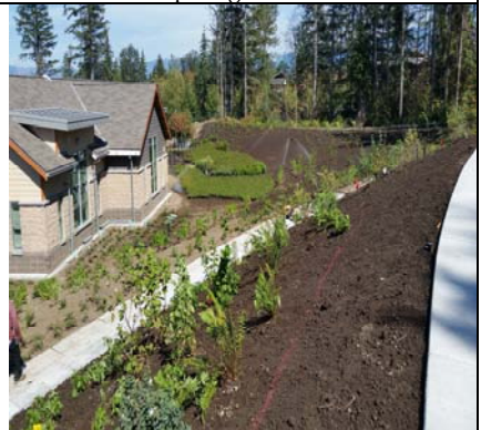
Trees And Shrubs Installation In Process
