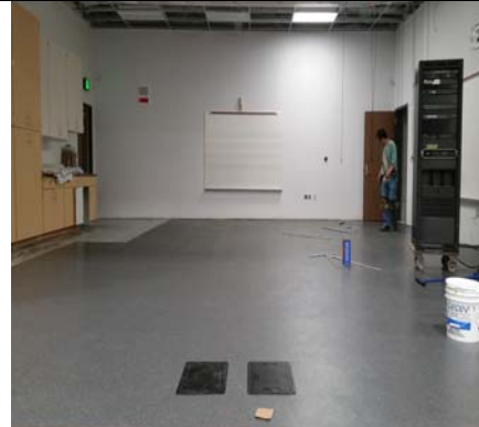
Stage Flooring/Floor Box Completion
