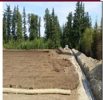
Underground Electric & Telecom Lines
