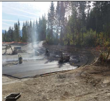
Asphalt Treated Base At Parking Lot
