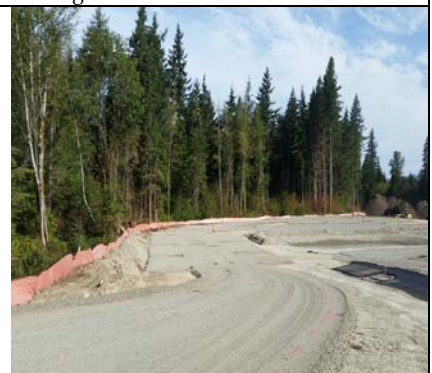
Crushed Rock Underlayment At Entry
