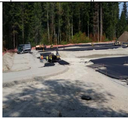
Crushed Rock & ATB At Bus Loop
