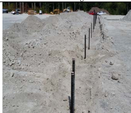
Under Building Slab Plumbing
