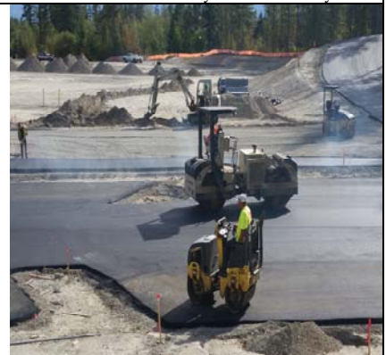
Compacting The Asphalt Treated Base
