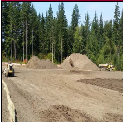
Topsoil Pile Continues To Get Smaller
